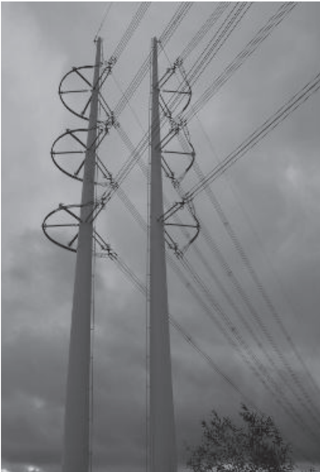
Stralingsarme Wintrackmasten © L.J. Smale, Leiden
